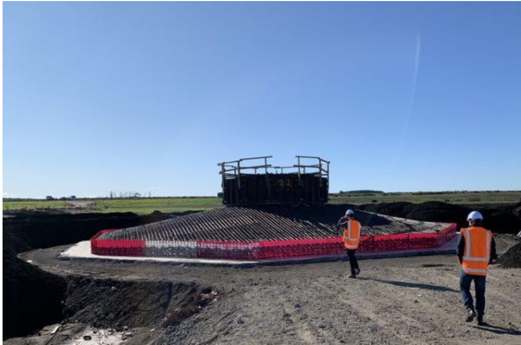
FIGURE 3 EXAMPLE OF FOUNDATION CAGE PRIOR TO POURING
