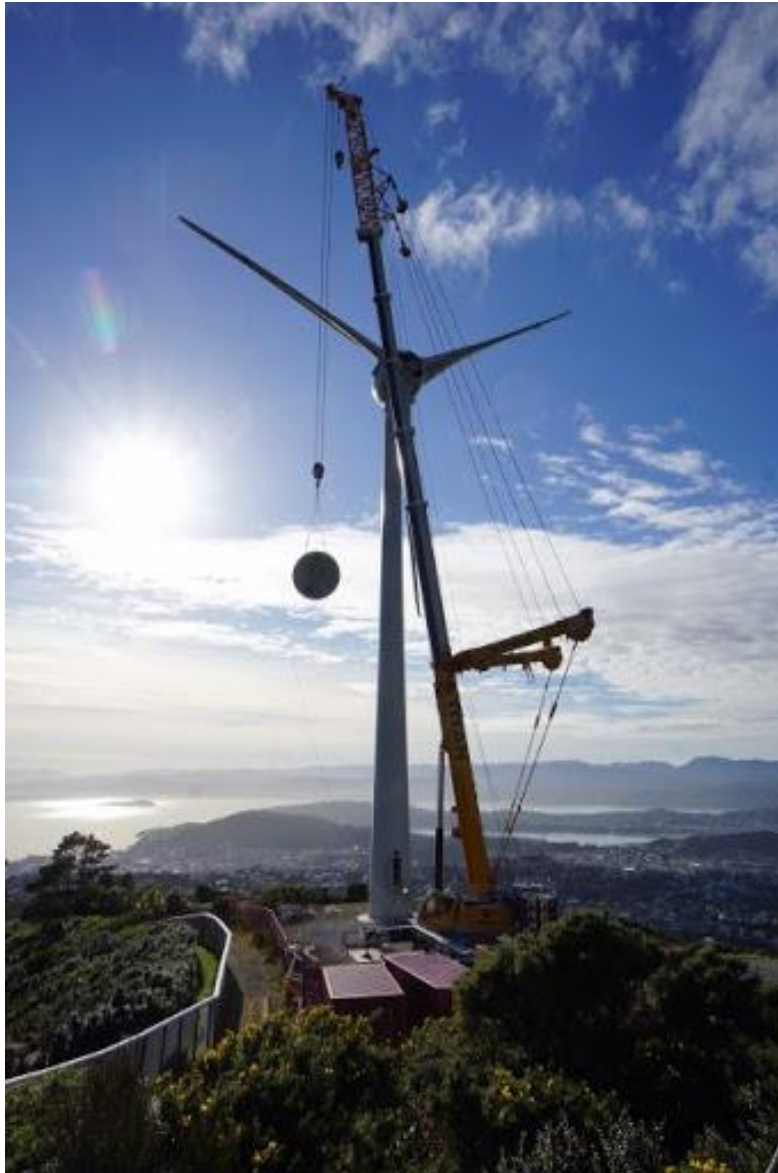
FIGURE 6 EXAMPLE OF TURBINE ERECTION CRANE
