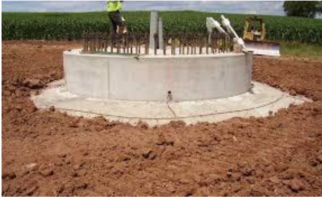
FIGURE 5 EXAMPLE OF A FOUNDATION AFTER BACK FILLING
