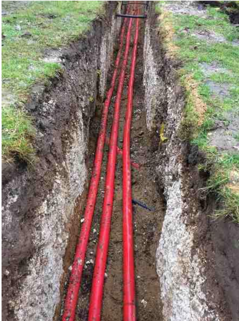
FIGURE 7 EXAMPLE OF HV CABLES IN CABLE TRENCH BEFORE BACKFILLING
