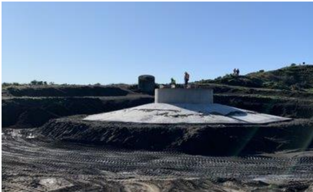
FIGURE 4 EXAMPLE OF FOUNDATION AFTER POURING
