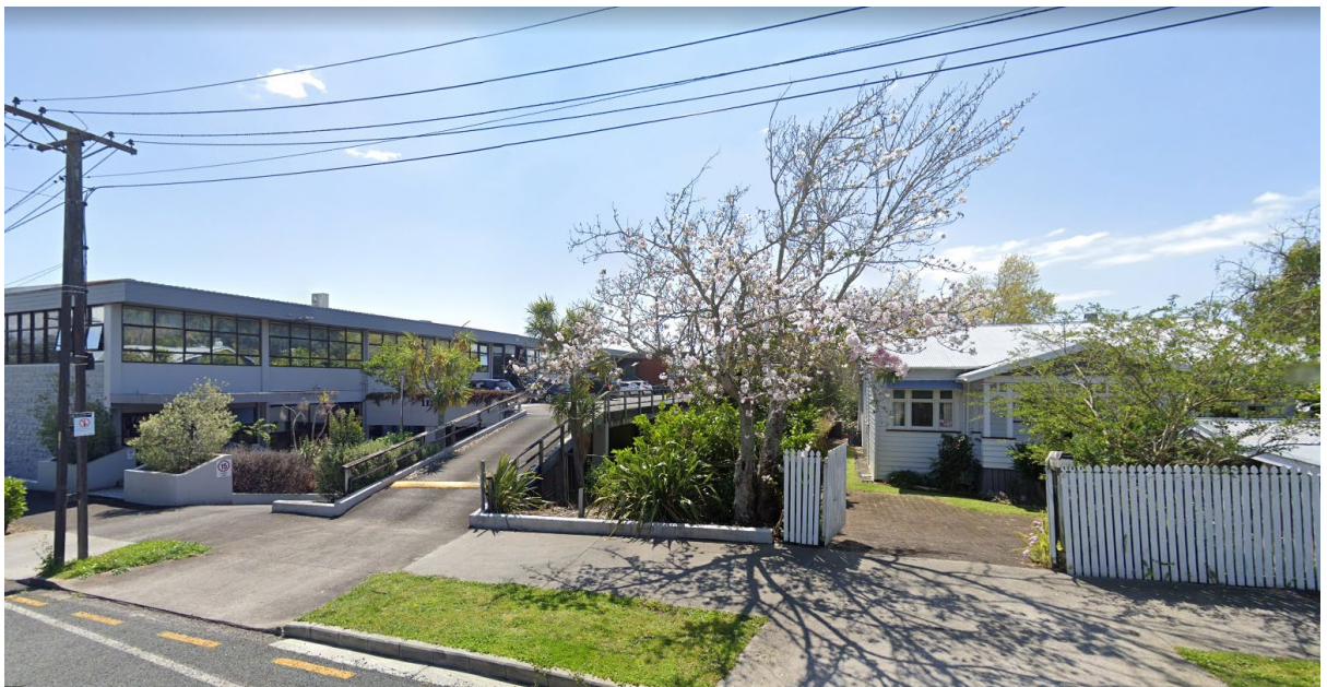
Figure 2: Google Street View image looking from Grange Road to the boundary interface of 111 Grange Road
